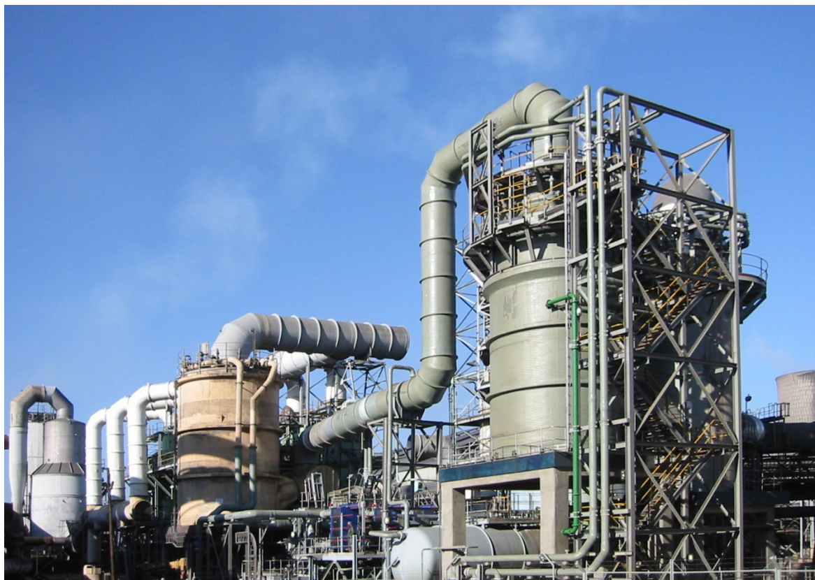
Pic. 3: Cleaning off gases by means of absorption and aerosol removal downstream of pyro-metallurgical processes in non-ferrous industries.
