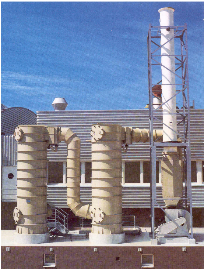
Pic. 6: Scrubbing plant for the absorption of noxious gas components and the removal of acidic mists and salt aerosols downstream of multiple-hearth furnaces for the production of inorganic raw chemicals
