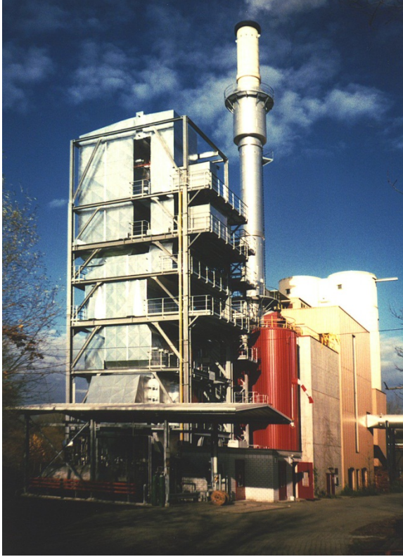
Pic. 10: SCR process for a retrofitted unit in the municipal waste incineration. Low dust denitrification of the flue gases.
