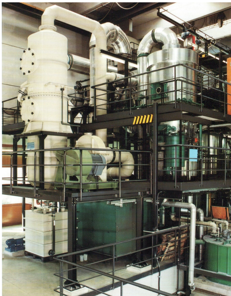
Pic. 8: Gas Cleaning Plant downstream a clinical waste incineration using PTA-Technology
