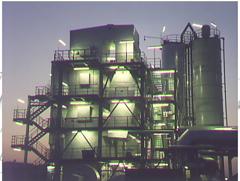
Pic. 11: Separation of dust removal, adsorption and neutralization of noxious substances incl. The elimination of Dioxins/Furans, CO and Hg.
